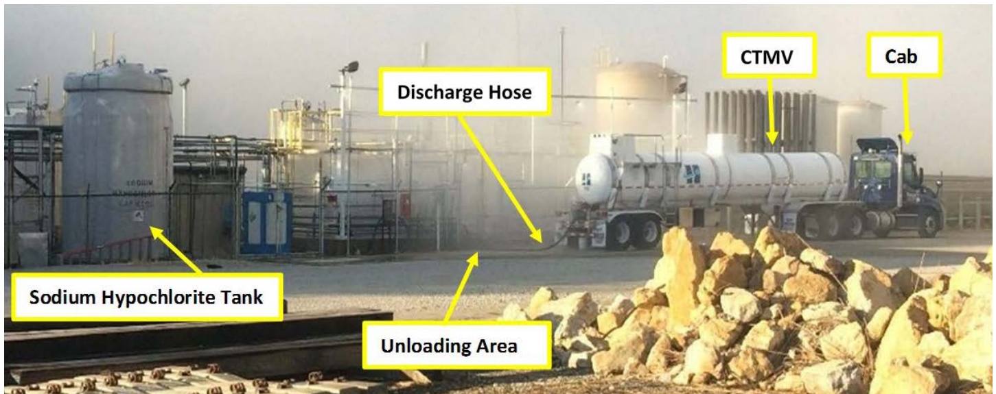
Figure 15. Post-incident photograph of Harcros CTMV connected to sodium hypochlorite fill line at Mod B unloading area, showing sodium hypochlorite tank and cab of CTMV (Source: MGPI).
