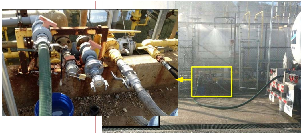
Figure 4. Chemical unloading operations at the time of the incident (Source: MGPI). 6
